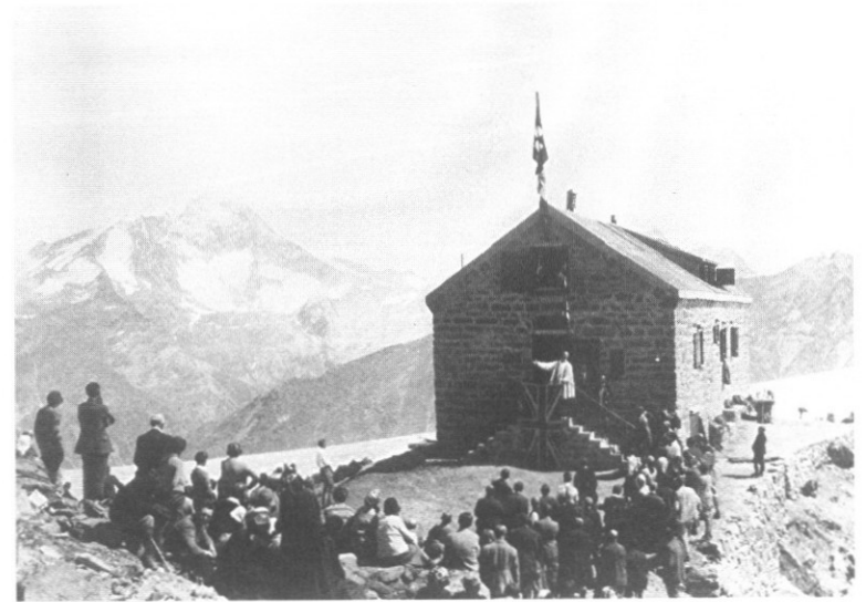
The Rededication of the Enlarged Britannia Hut
